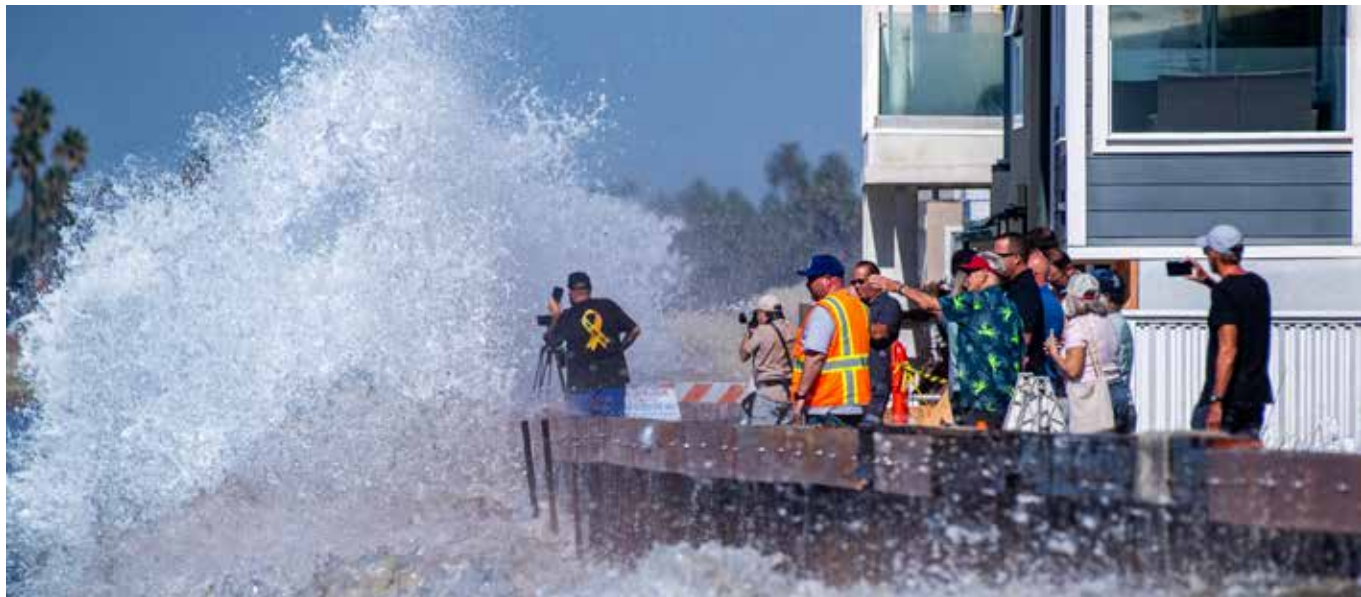
Locals and members of the media fill the boardwalk as king tides slam the wooden bulkhead on the Peninsula in Long Beach, Monday, Sept. 28, 2026.
