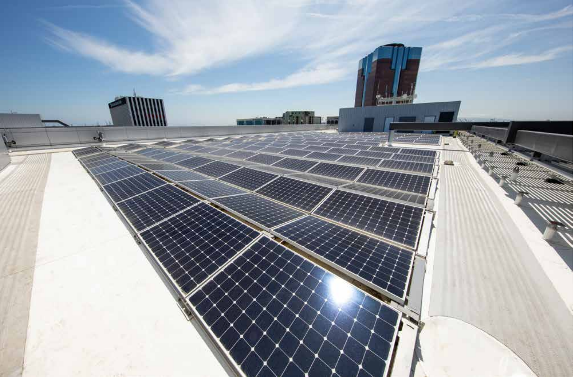
City Hall’s solar array will produce approximately 140 kilowatts of power. (Fukushima Photography)
