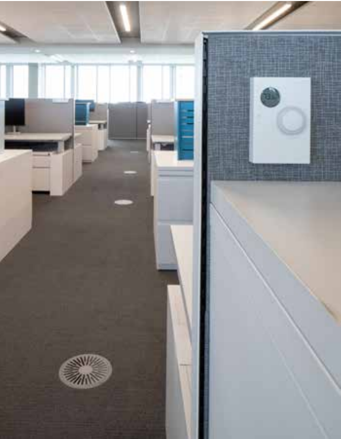
The underfloor HVAC system includes controllable dials for every workspace grouping so employees can set the temperature around their desks. (Fukushima Photography)
