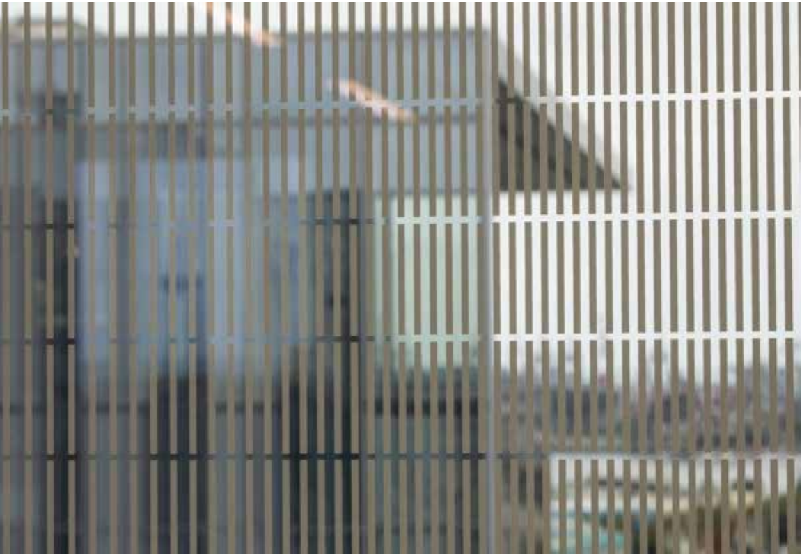
The window fritting on City Hall’s south side is placed close together on the right sides of the windows to block out heat while still letting in daylight. (Fukushima Photography)
